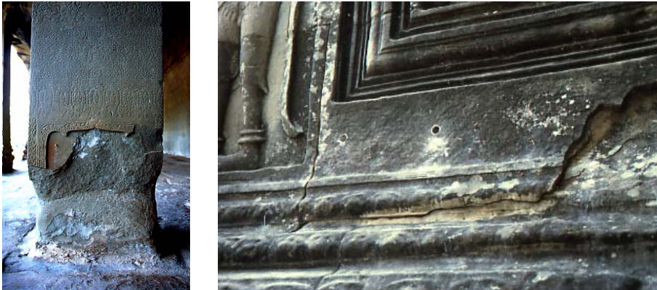
Fig. 4 a, b: Pillar from the northern gallery of the third enclosure (a, left) and surface with contour scalings (b, right)
